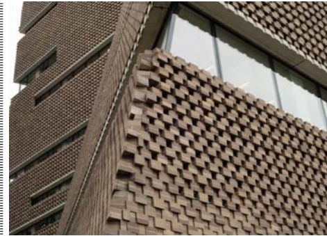
Tate Modern's extension, Londres, 2016, Herzog & de Meuron : https://www.dezeen.com/2016/06/20/tate-modern-switch-house-herzog-de-meuron-london-opens-to-the-public-jim-stephenson/
