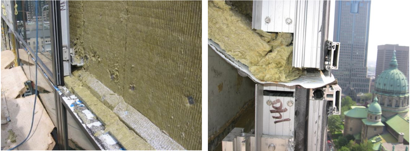
Figure 9: Curtain wall cladding at parapet level.
