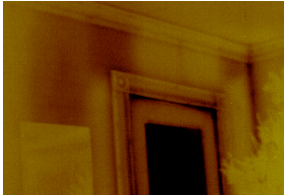
Image 4. Properly installed cellulose is an excellent insulation. Unfortunately it is often poorly installed with missed areas and settling the most common quality problems.
