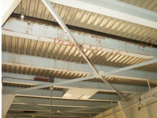
Figures 2 and 3. Photos showing signs of water ingress below roof deck (at left) and signs of roof membrane deterioration above
