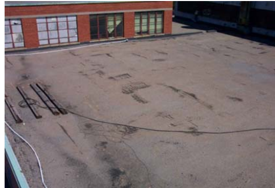
Figures 2 and 3. Photos showing signs of water ingress below roof deck (at left) and signs of roof membrane deterioration above
