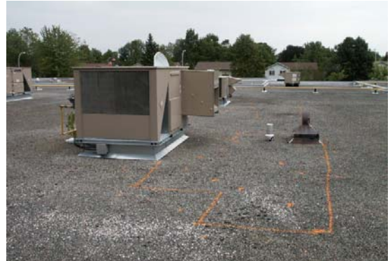
Figures 6 and 7. Typical infrared scan of wet area within roofing system at left. At right, paint typically used on roof surface to delineate suspect area of roofing system.
